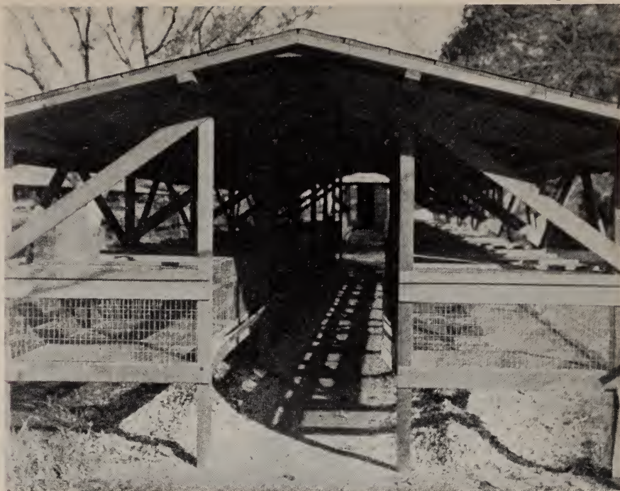
Fig. 37. An orchard poultry house which is in use today, showing construction similar to that shown in figure 36.
